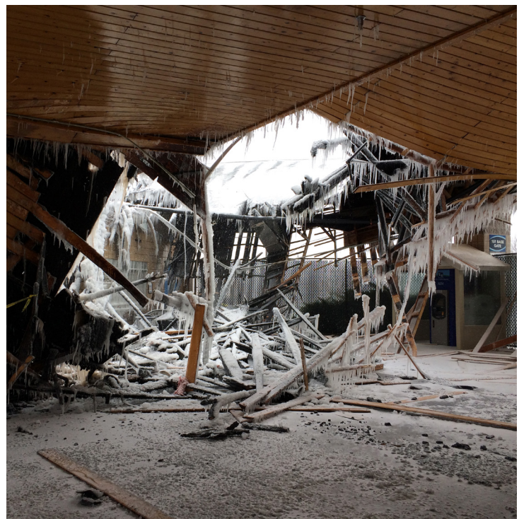
First base concourse
